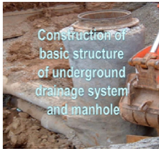
Fig. 2. 2: Construction of underground drainage system.
