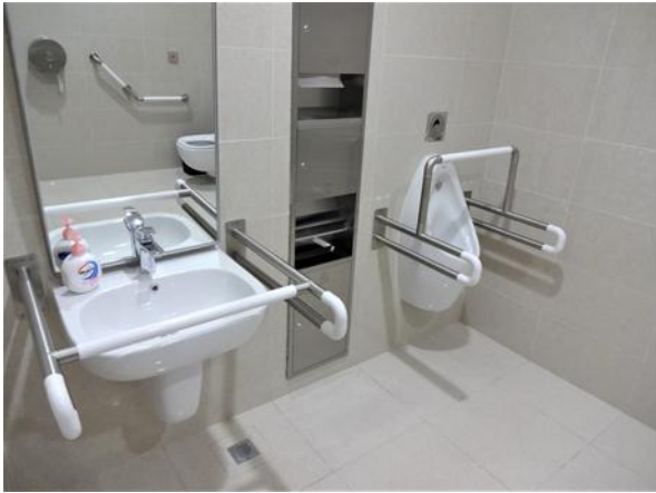
Photo45. Inside the bathroom of the high-speed railway station 2
