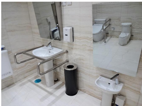
Photo33. Inside of the multipurpose bathroom at subway station2
