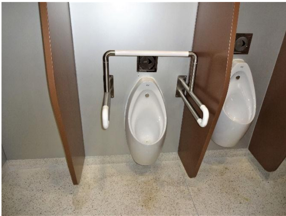
Photo46. Urinals for men toilet in the high-speed railway station
