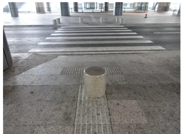
Photo49. Outside the building2
