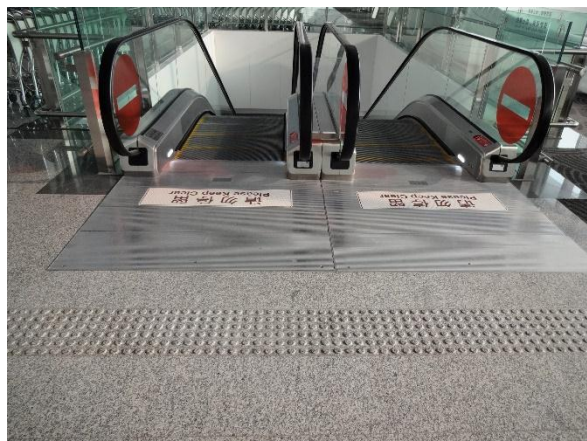
Photo5. Guidance blocks in front of escalators
