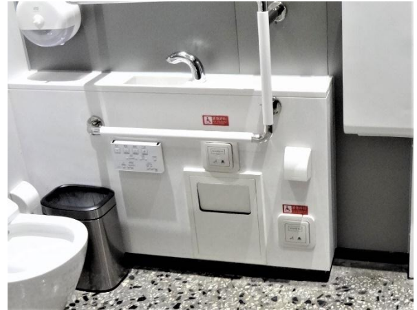
Photo16. Equipment of multipurpose bathroom 3
