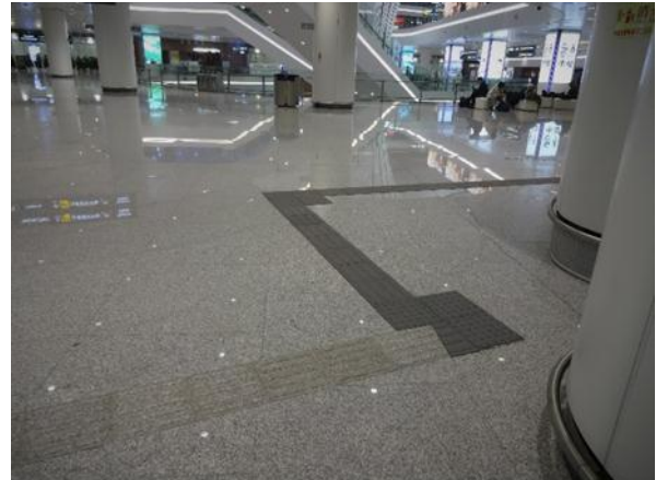
Photo9. Guidance blocks installed on the third floor
