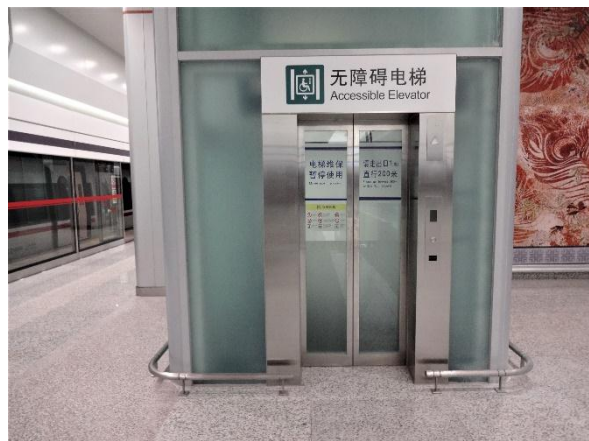
Photo42. elevator on the platform level
