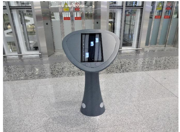
Photo17. Equipment to centrally control three elevator cars at once
