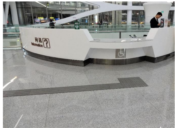
Photo10. Blocks leading to the information booth
