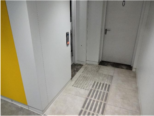
Photo57. Multipurpose bathroom in the parking lot
