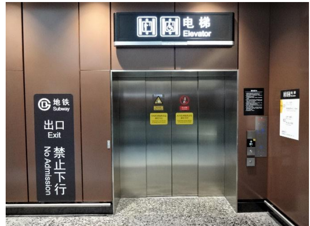
Photo28. Elevator of the subway station (first basement level)
