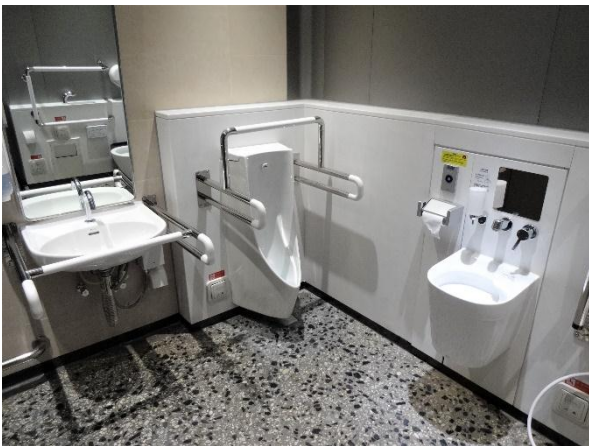
Photo15. Equipment of multipurpose bathroom 2
