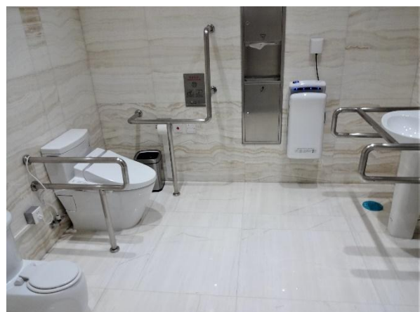
Photo32. Inside of the multipurpose bathroom at subway station 1
