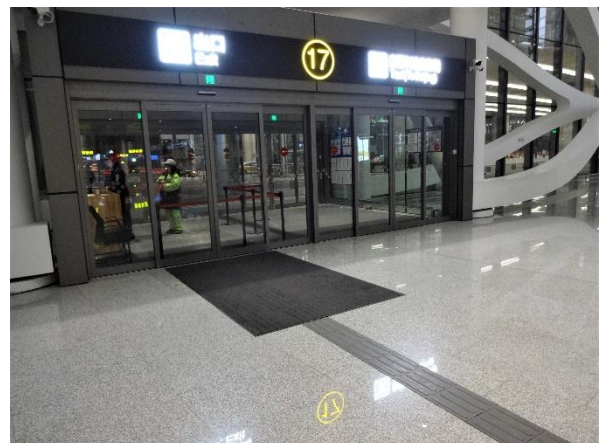
Photo11. Blocks at entrance/exit
