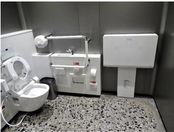
Photo14. Equipment of multipurpose bathroom 1
