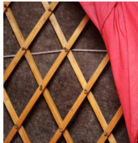
Fig 4. Kerege – a rope, folding lattice walls and a large piece of felt covering the structure
