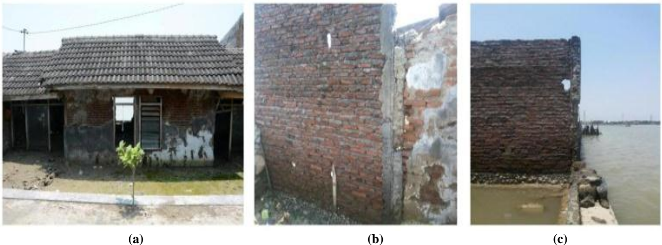
Fig 3. Situation of the site: (a) a house that directly adjacent to the sea; (b) the broken part of clay brick masonry wall; (c) the area outside the house that submerged by seawater and routine tidal flooding
