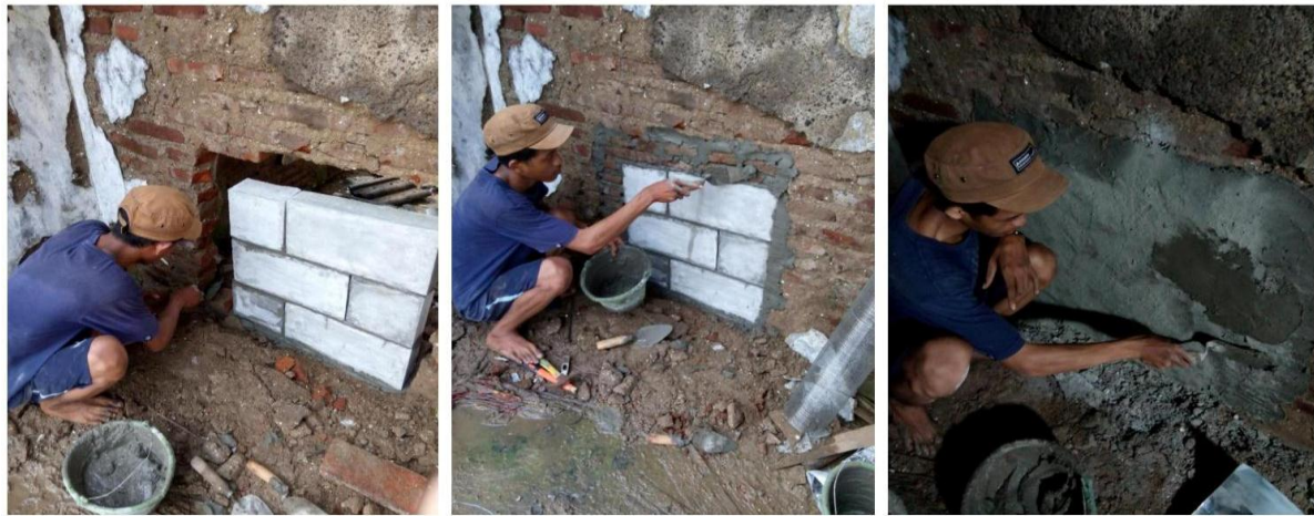
Fig 9. Retrofitting of masonry wall in site – (a) Filling the removed part by concrete bricks; (b) filling the space between new concrete bricks and the old masonry wall; (c) Plastering the retrofitted masonry wall
