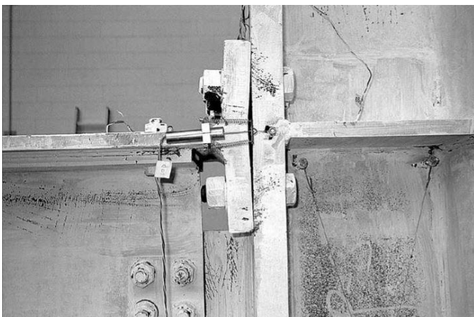
Fig 4. Failure mode of tested steel connection [25]
