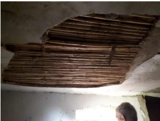
Figure 11. Ceiling of a room at Tighremt Ait Louakhoumi / photo taken in October 2018
