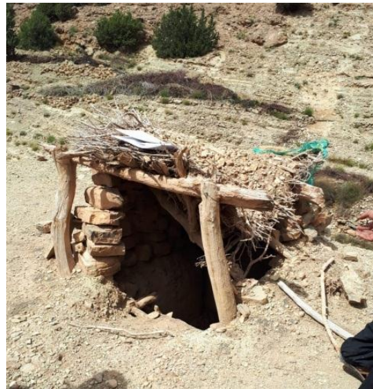
Figure 12: Edicule allowing access to the terrace, Tghremt Ait Louakhoumi
