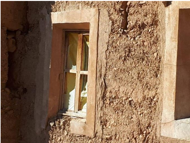
Figure 10. Windows added and modified / photo taken in October 2018
